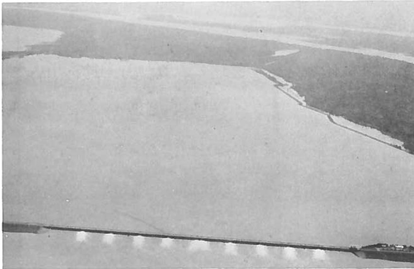
Figure 3. Morganza Spillway in operation during the 1973 flood.
